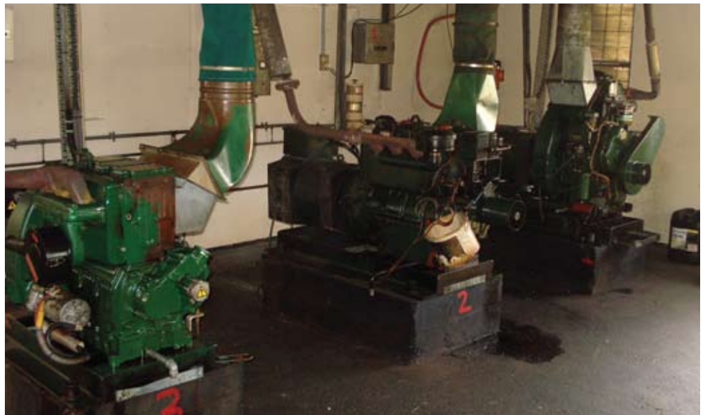
Figure 24. The three Lister diesel generators
