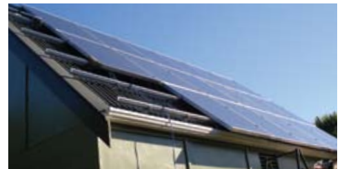
Figure 25. The PV array being installed on a framing system
