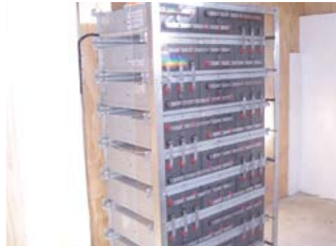
Figure 9. The 48v battery bank
