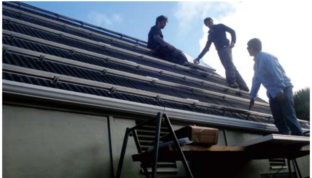
Figure 5. PV array framing being installed on a roof on Mana Island
