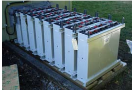
Figure 1. A battery bank installed on a concrete base, with the enclosure removed
