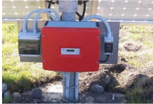
Figure 4. An inverter installed on the PV system on Little Barrier Island
