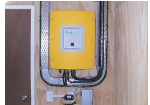
Figure 10. The Sunny Island inverter
