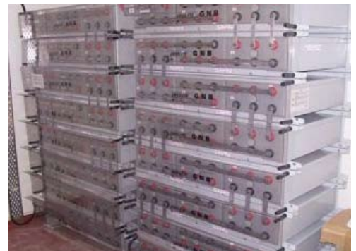
Figure 16. The two 48V battery banks
