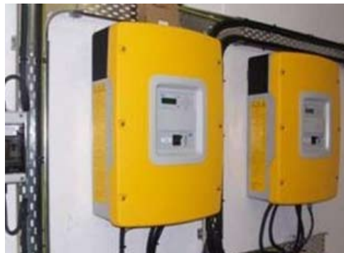
Figure 15. The two Sunny Island inverters
